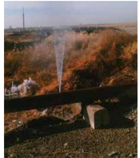
Water infrastructure in SEE requires significant investment
