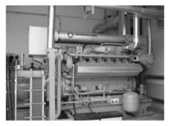
Figure 4.19 Co-generator run on biogas (www.cogen3.net)
