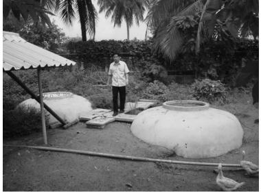
Figure 4.6 Fixed-dome digesters treating piggery wastewater, central Thailand
